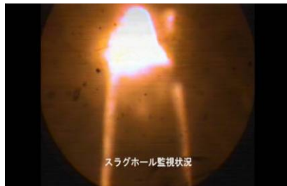
Slag hole view from lower side 煤渣从煤渣孔落下
